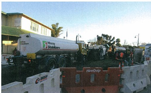
Foam Bitumen Stabilising Train
