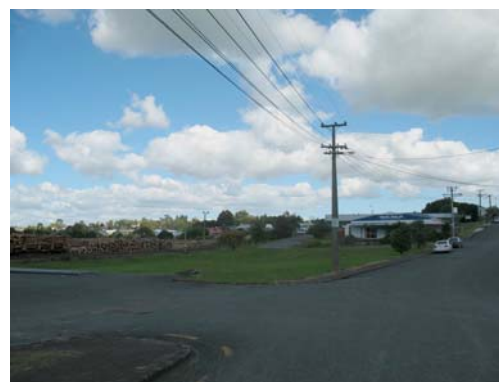
Station Road before
