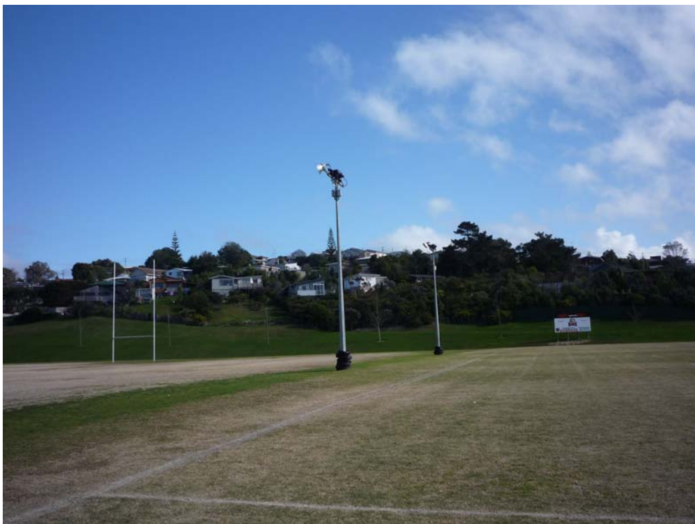
Figure 3: Site photograph of two of the existing floodlight towers.
