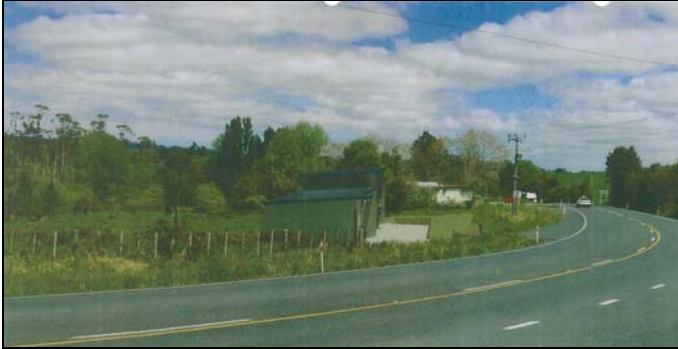
Figure 7 - Prior to landscaping being implemented
