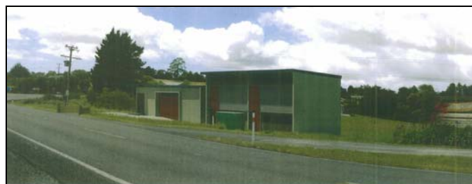
Figure 5 – Prior to landscaping being implemented
